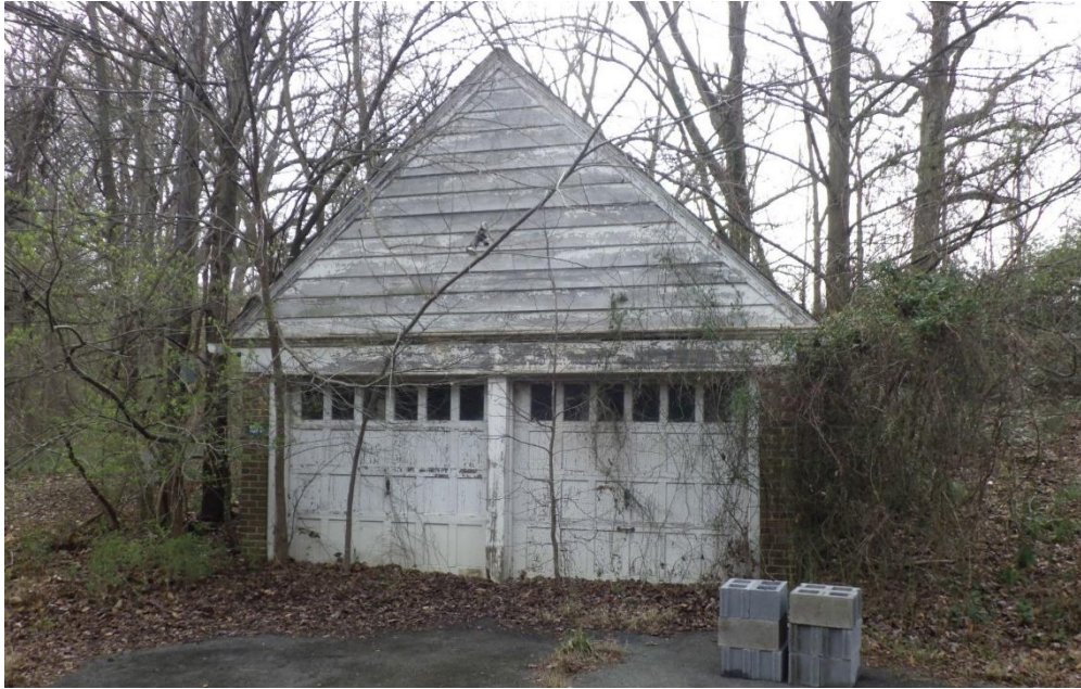
Figure 8-36: Building 1071 – Facing south, location shown on Appendix A, Figure 3
