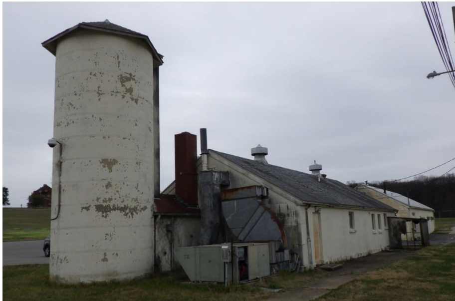
Figure 8-49: Building 1002 facing east, location shown on Appendix A, Figure 3
