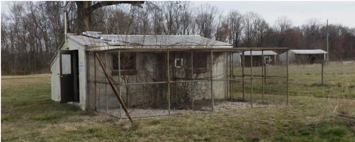
Figure 8-46: Building 1329 – Facing north, location shown on Appendix A, Figure 3
