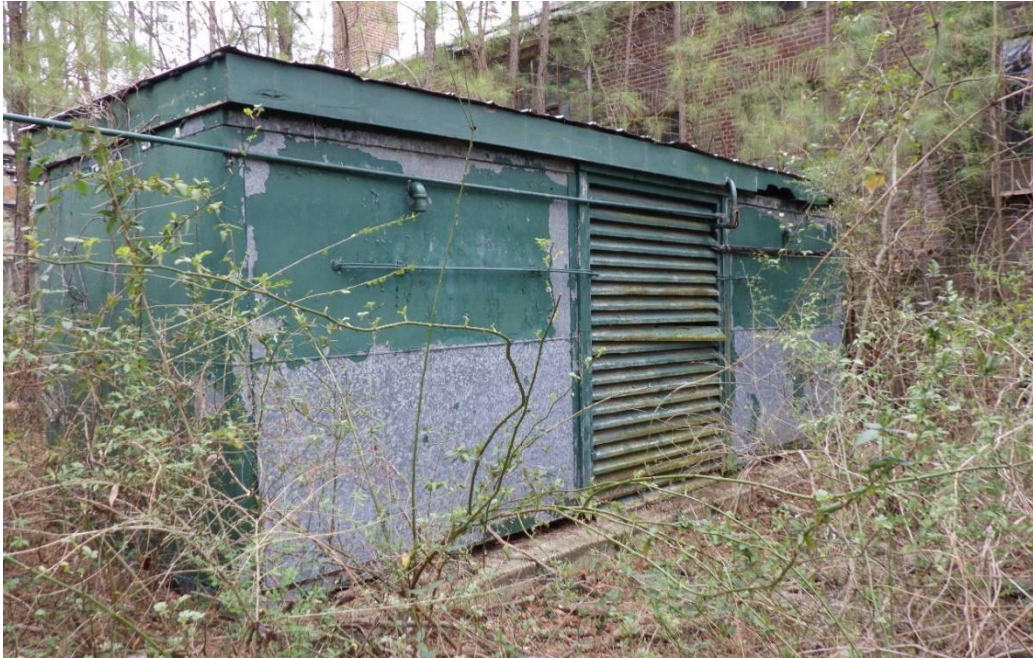
Figure 8-29: Building 488, facing northwest, location shown on Appendix A, Figure 3
