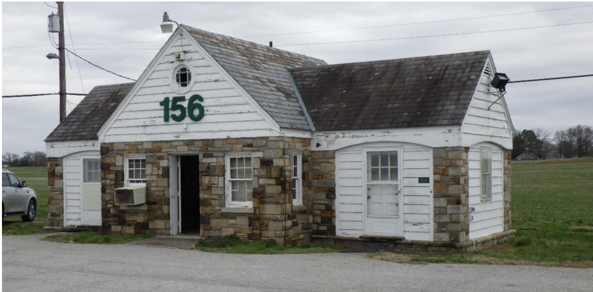
Figure 8-9: Building 156, facing southeast location shown on Appendix A, Figure 3
