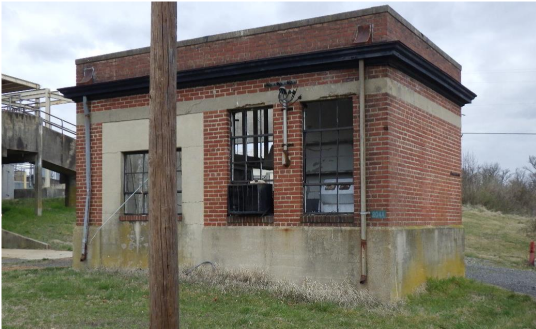
Figure 8-4: Building 204A, facing northwest, location shown on Appendix A, Figure 3
