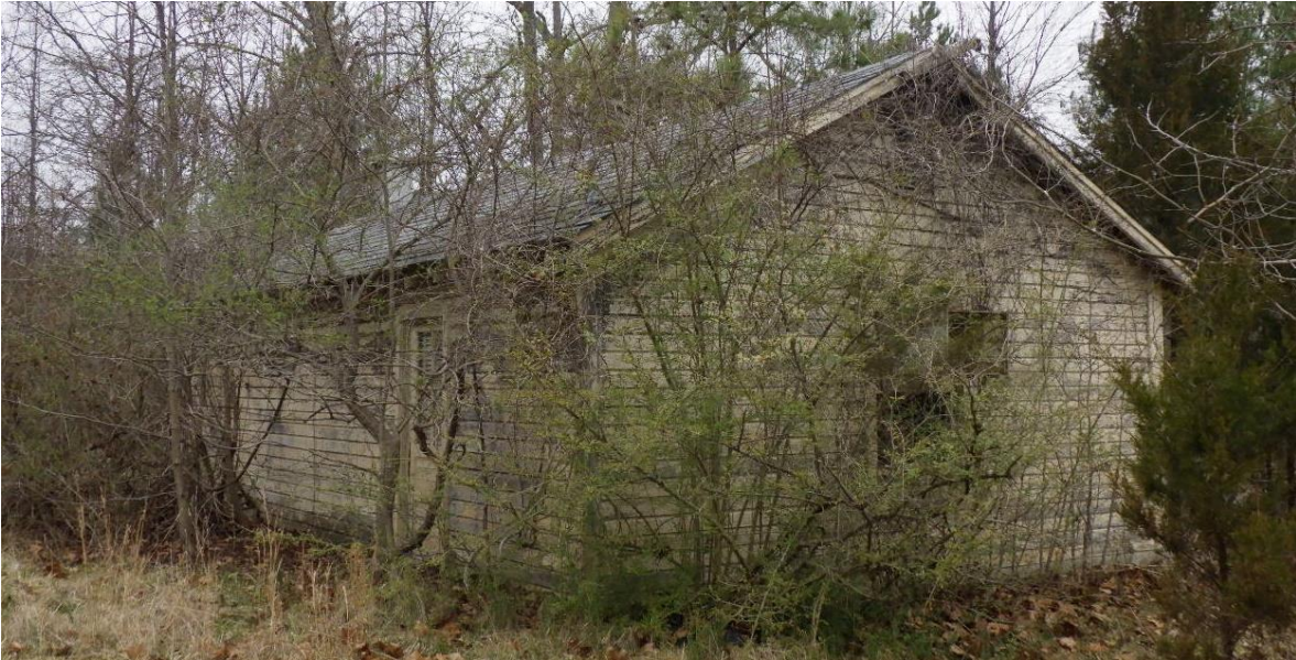
Figure 8-11: Building 468, facing northwest, location shown on Appendix A, Figure 3
