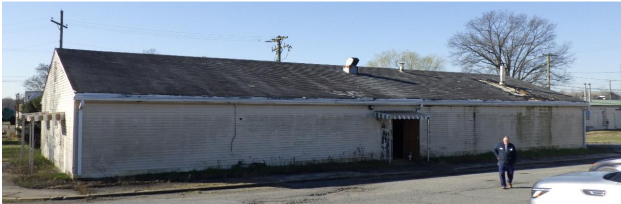
Figure 8-3: Building 177B, facing southwest, location shown on Appendix A, Figure 3
