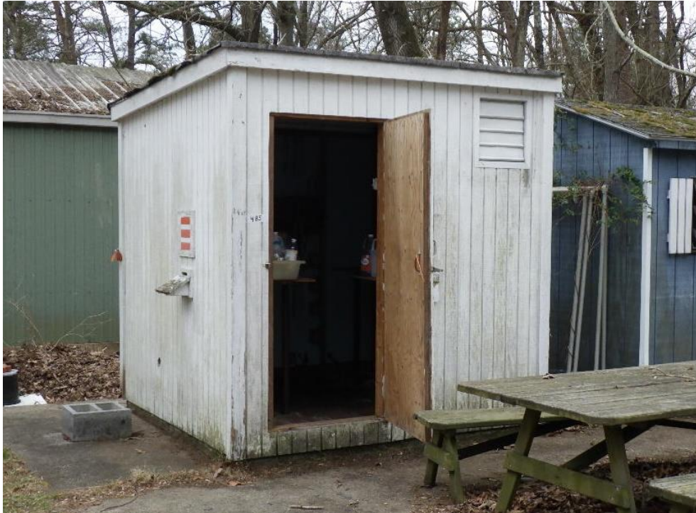
Figure 8-27: Building 485, facing south, location shown on Appendix A, Figure 3
