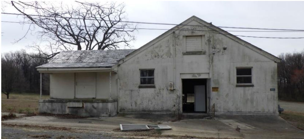
Figure 8-54: Building 1063 facing southeast, location shown on Appendix A, Figure 3
