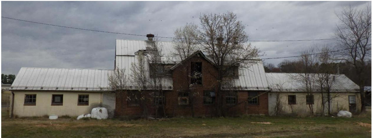
Figure 8-18: Building 434 view from south, location shown on Appendix A, Figure 3
