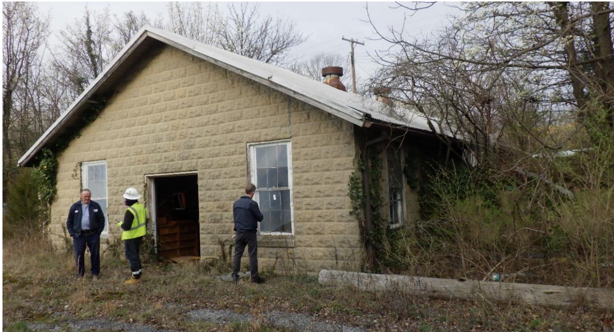
Figure 8-3: Building 40, facing southwest, location shown on Appendix A, Figure 2
