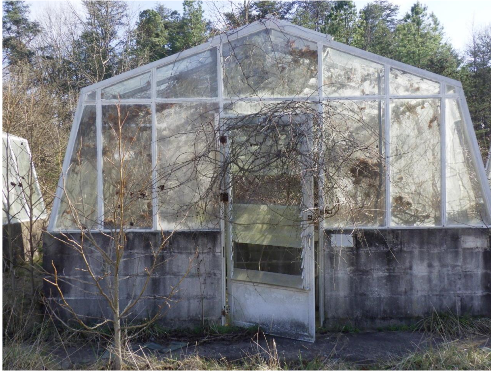
Figure 8-16: Building 470EE, facing south, location shown on Appendix A, Figure 3
