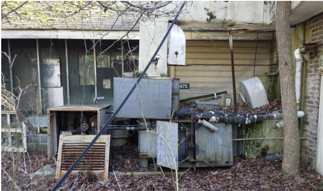
Figure 8-25: Building 475, facing southeast, location shown on Appendix A, Figure 3
