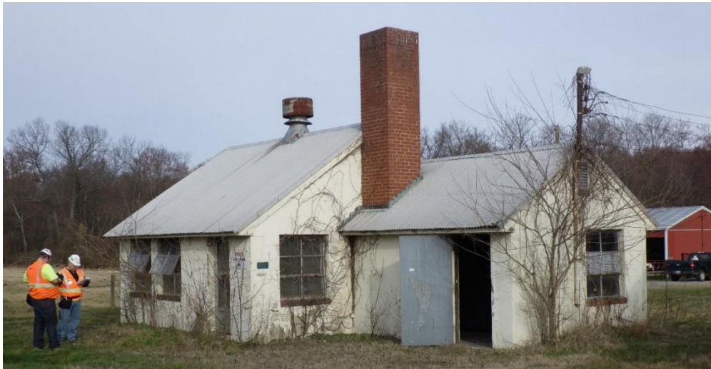
Figure 8-44: Building 1292 – Facing northwest, location shown on Appendix A, Figure 3
