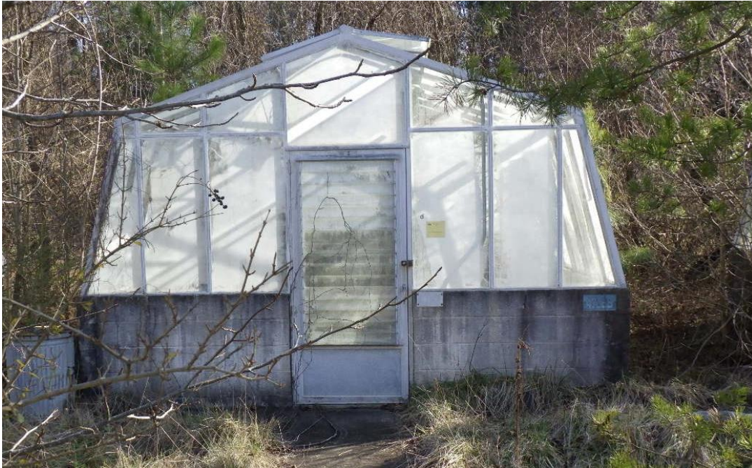
Figure 8-13: Building 470BB, facing south, location shown on Appendix A, Figure 3
