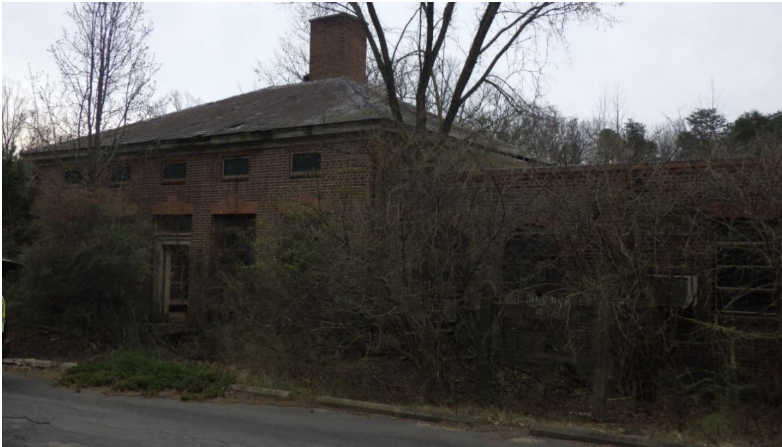
Figure 8-23: Building 470, facing southeast, location shown on Appendix A, Figure 3
