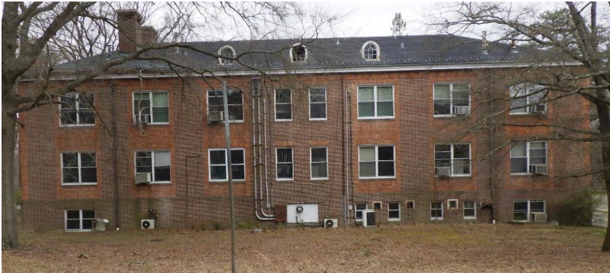
Figure 8-26: Building 476, facing east, location shown on Appendix A, Figure 3
