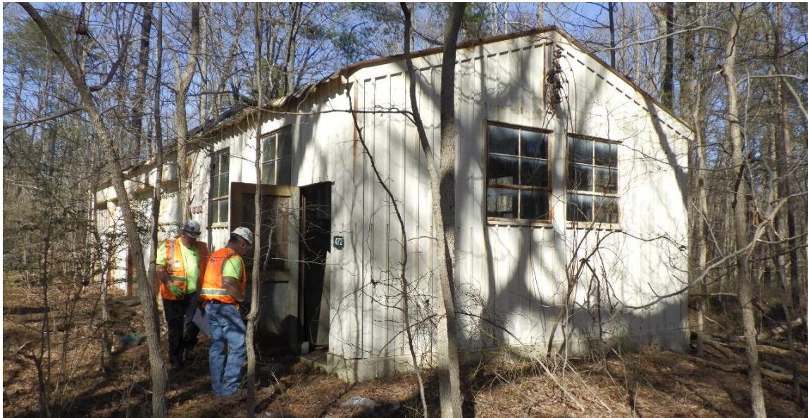
Figure 8-22: Building 472, facing north, location shown on Appendix A, Figure 3
