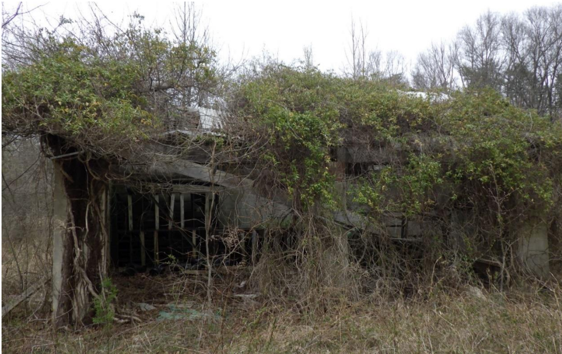
Figure 8-35: Building 543A, facing south, location shown on Appendix A, Figure 4
