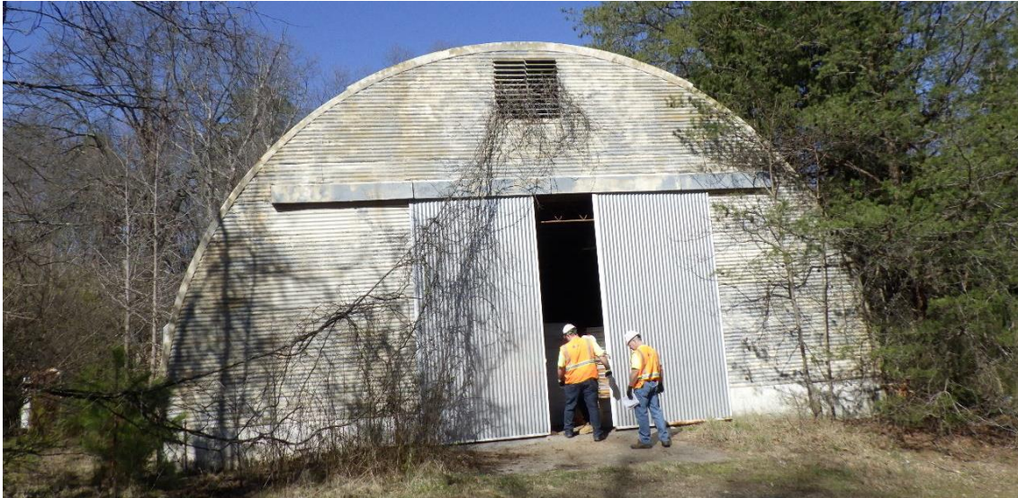
Figure 8-24: Building 470B, facing north, location shown on Appendix A, Figure 3
