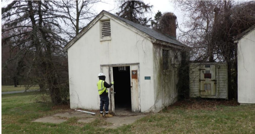
Figure 8-51: Building 1052 facings Southwest, location shown on Appendix A, Figure 3
