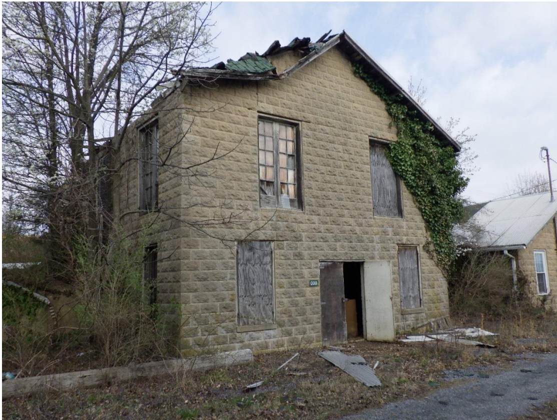
Figure 8-2: Building 39, facing northwest, location shown on Appendix A, Figure 2
