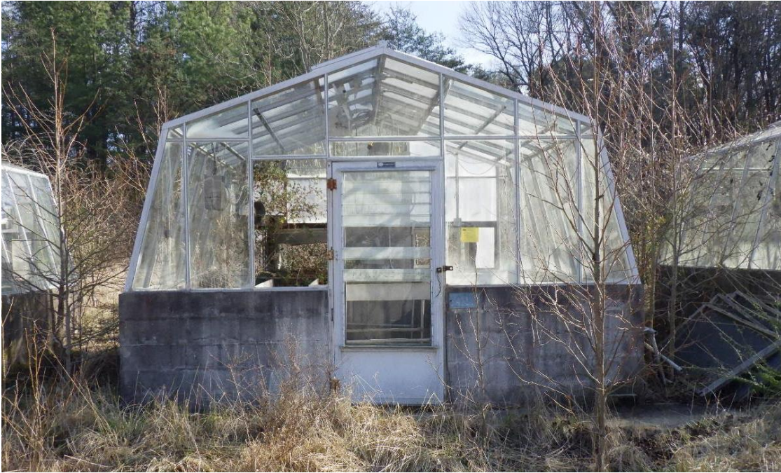
Figure 8-20: Building 470II, facing south, location shown on Appendix A, Figure 3
