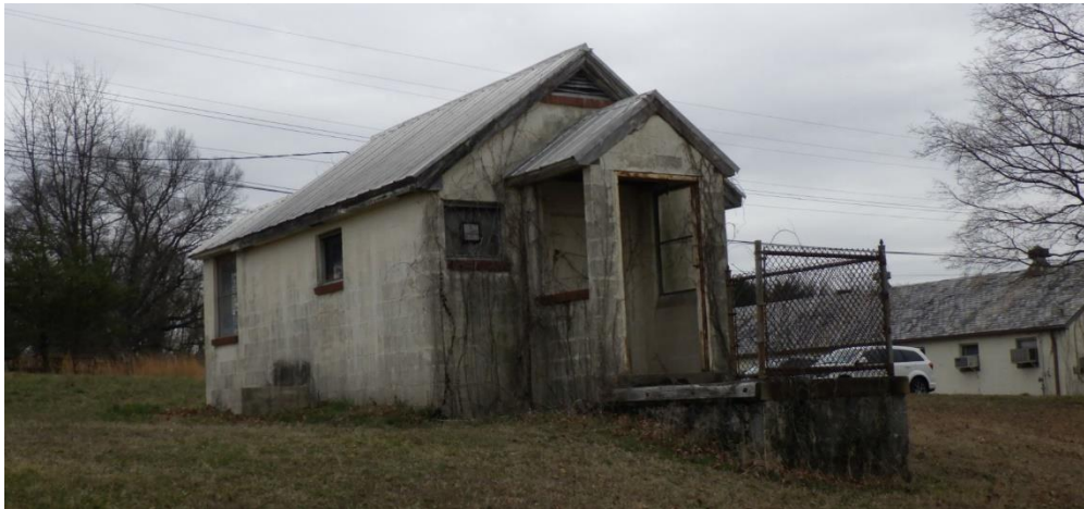
Figure 8-39: Building 1104 – Facing south, location shown on Appendix A, Figure 3
