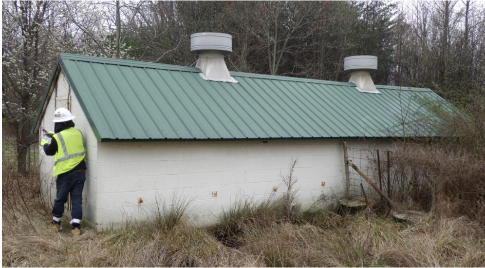
Figure 8-33: Building 541D, facing southeast, location shown on Appendix A, Figure 4 ACM
