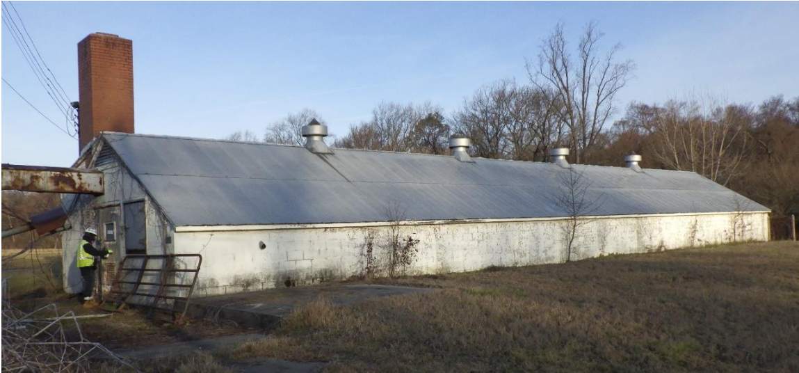
Figure 8-48: Building 1425 – Facing northwest, location shown on Appendix A, Figure 3 ACM
