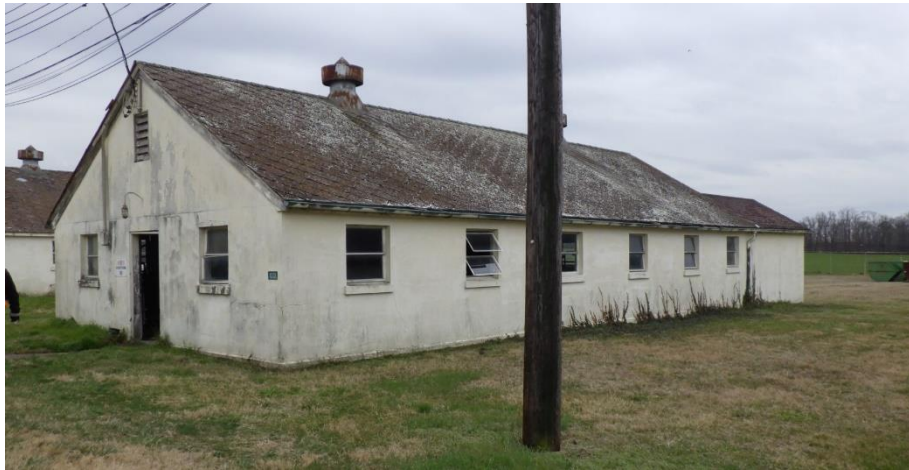
Figure 8-50: Building 1005 facing southwest, location shown on Appendix A, Figure 3
