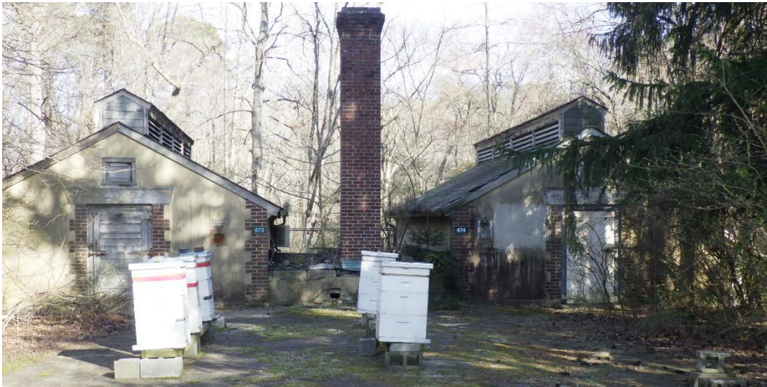
Figure 8-23: Building 473 (on the left), facing east, location shown on Appendix A, Figure 3 ACM
