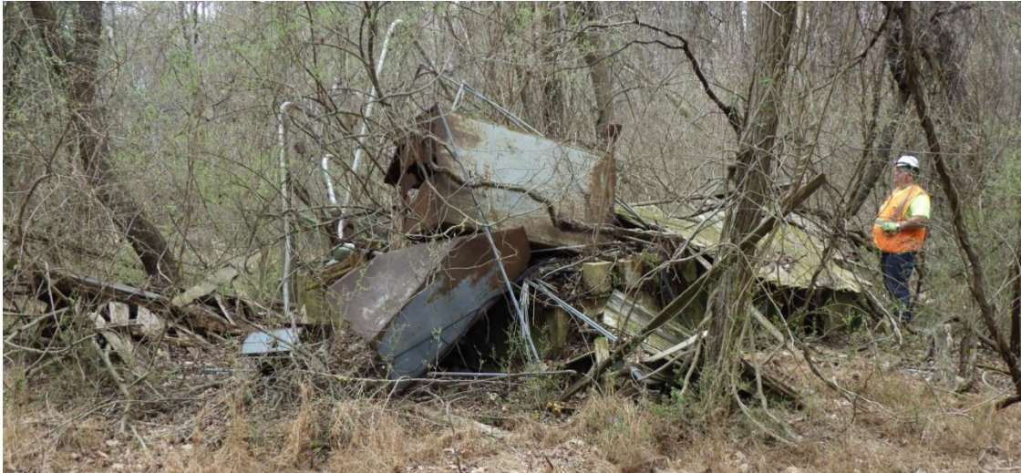
Figure 8-9: Building 452, facing north, location shown on Appendix A, Figure 3
