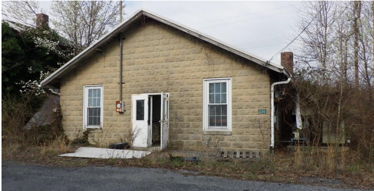
Figure 8-1: Building 38, Facing west, location shown on Appendix A, Figure 2
