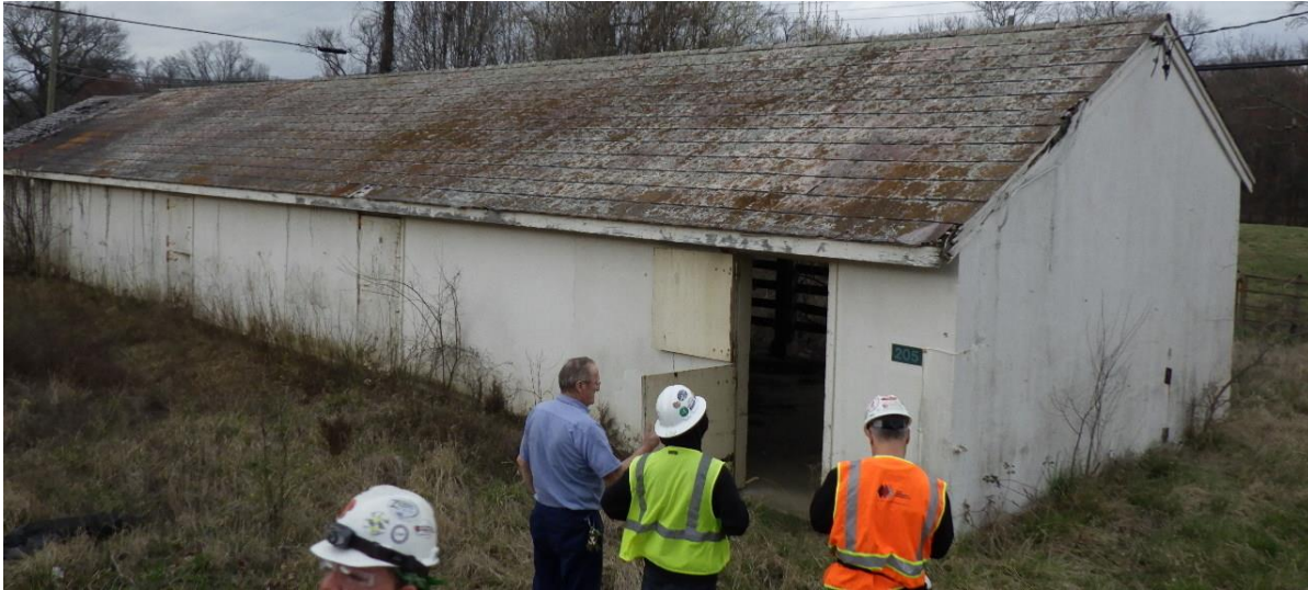
Figure 8-5: Building 205, facing northeast, location shown on Appendix A, Figure 3
