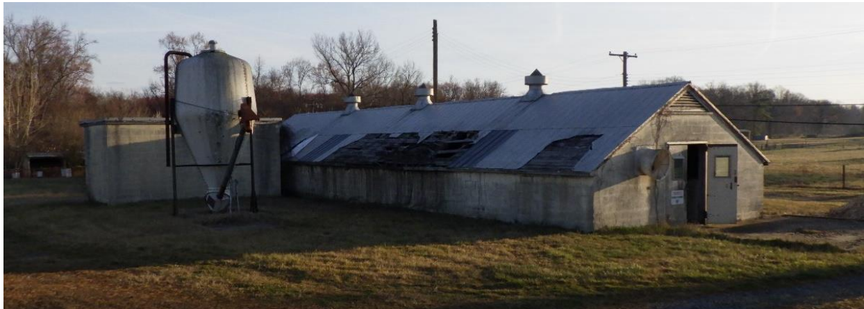
Figure 8-47: Building 1422 – Facing northwest, location shown on Appendix A, Figure 3 ACM
