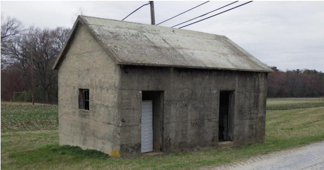
Figure 8-31: Building 524, facing northwest, location shown on Appendix A, Figure 4
