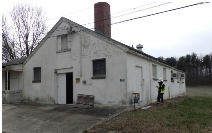
Figure 8-53: Building 1062 facing southeast, location shown on Appendix A, Figure 3
