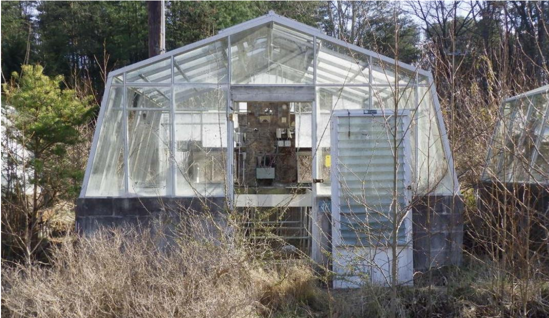
Figure 8-19: Building 470HH, facing south, location shown on Appendix A, Figure 3
