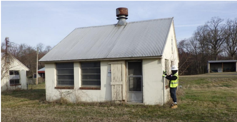
Figure 8-43: Building 1289 – Facing north, location shown on Appendix A, Figure 3
