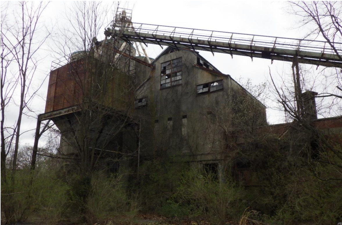
Figure 8-7: Building 85, facing southwest, location shown on Appendix A, Figure 3
