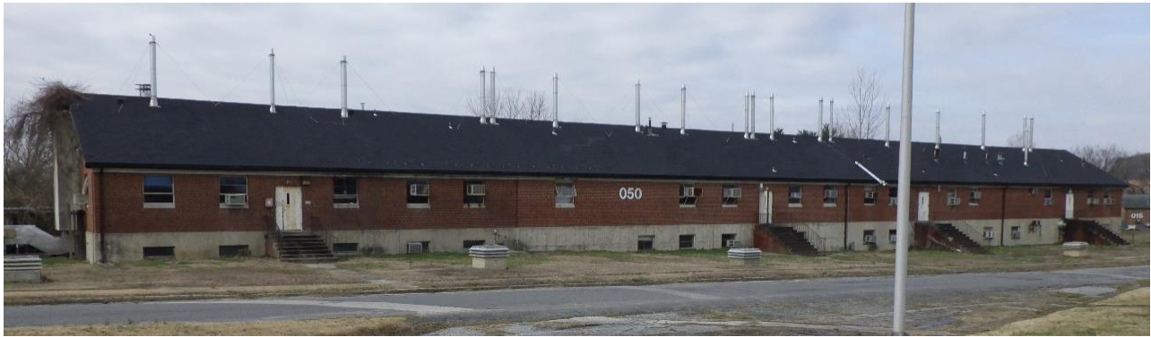
Figure 8-5: Building 50, facing southwest location shown on Appendix A, Figure 2
