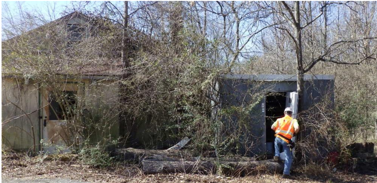
Figure 8-17: Building 327A, facing west, location shown on Appendix A, Figure 3
