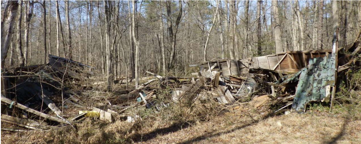
Figure 8-21: Building 471, facing north, location shown on Appendix A, Figure 3
