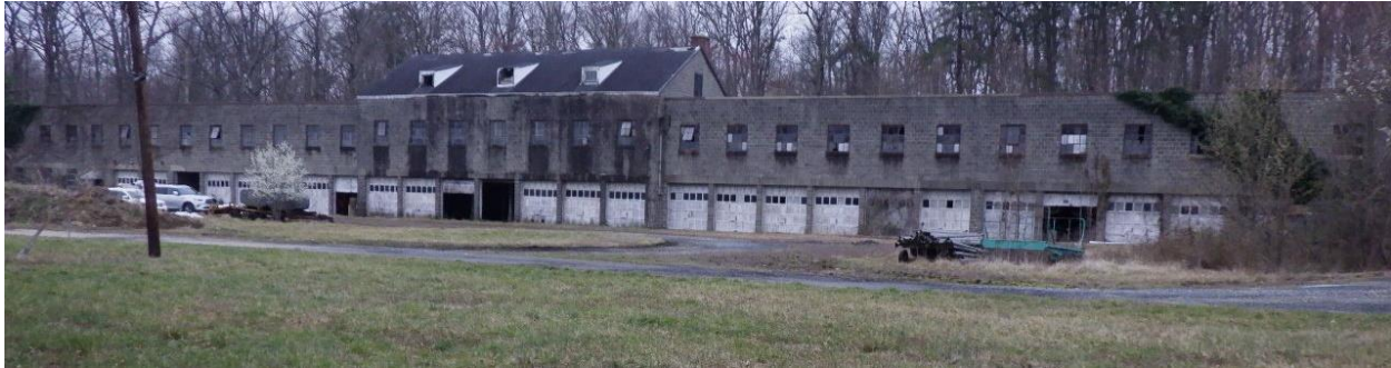
Figure 8-6: Building 60, facing southeast, location shown on Appendix A, Figure 2
