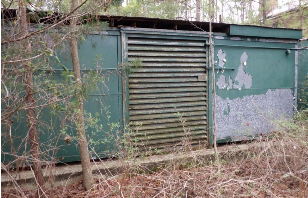
Figure 8-28: Building 487, facing northwest, location shown on Appendix A, Figure 3
