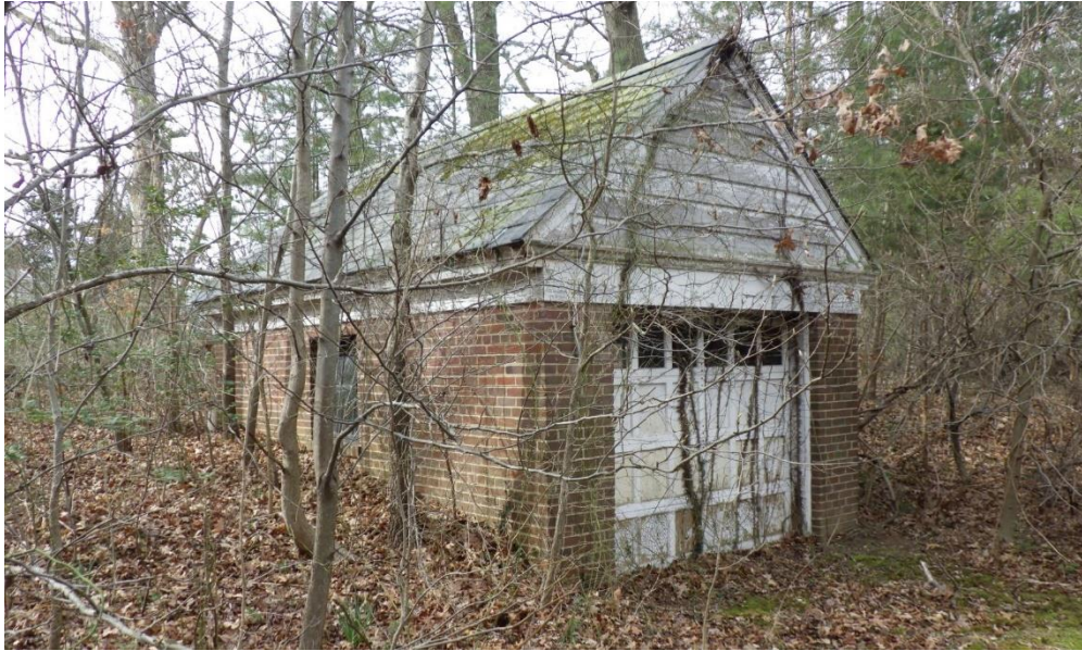
Figure 8-37: Building 1073 – Facing southwest, location shown on Appendix A, Figure 3
