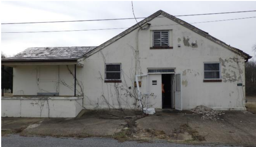
Figure 8-55: Building 1064 facing southeast, location shown on Appendix A, Figure 3
