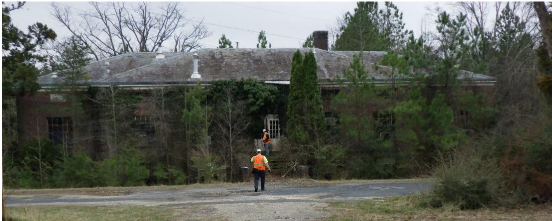
Figure 8-10: Building 467, facing south, location shown on Appendix A, Figure 3
