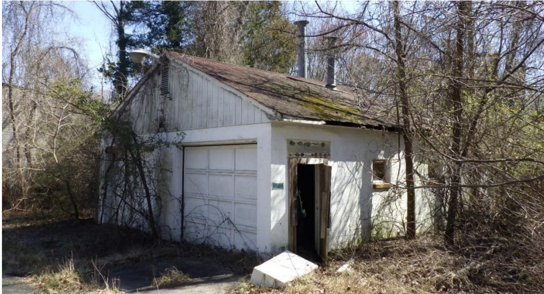
Figure 8-16: Building 288A, facing southeast, location shown on Appendix A, Figure 3
