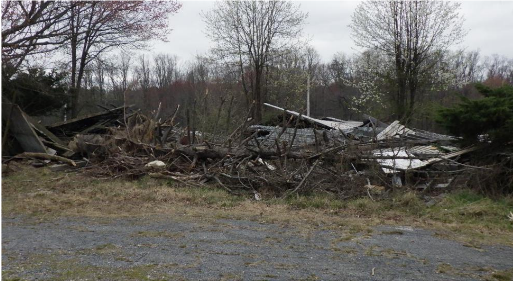
Figure 8-30: Building 506A, facing south, location shown on Appendix A, Figure 4
