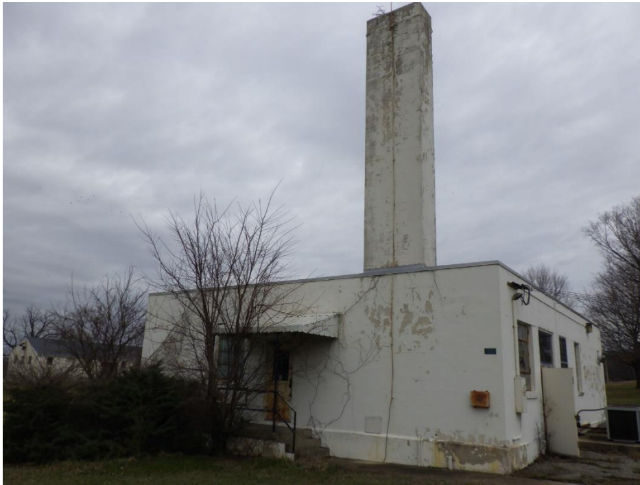
Figure 8-40: Building 1120 – Facing east, location shown on Appendix A, Figure 3
