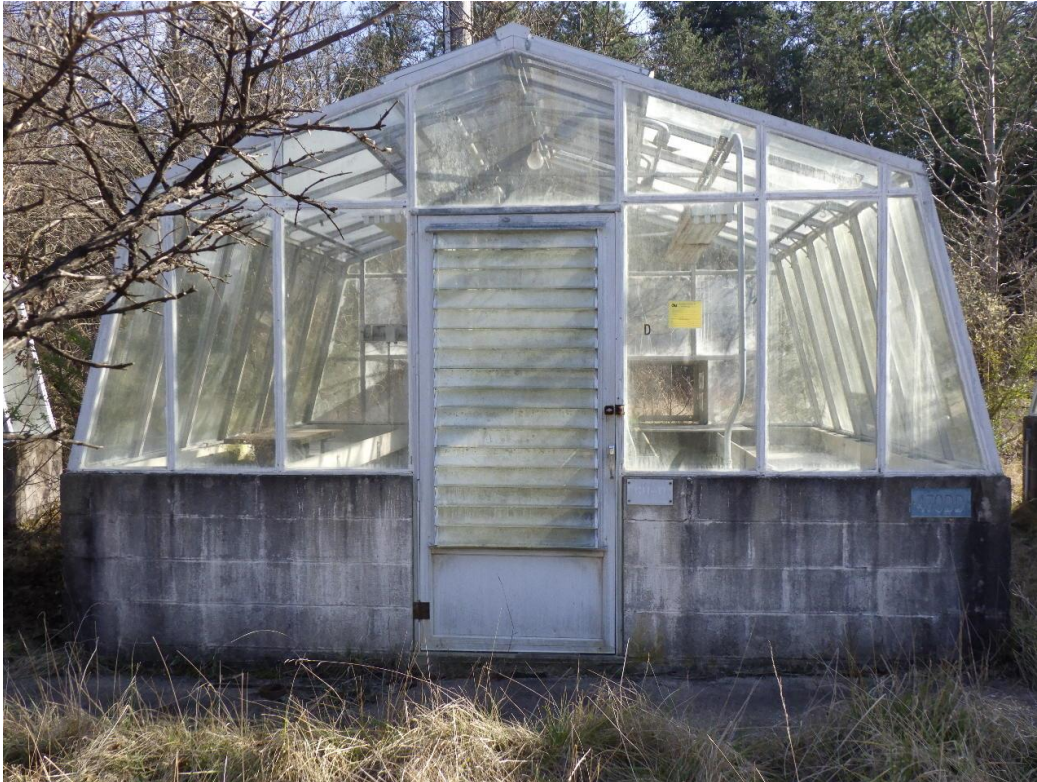
Figure 8-15: Building 470DD, facing south, location shown on Appendix A, Figure 3
