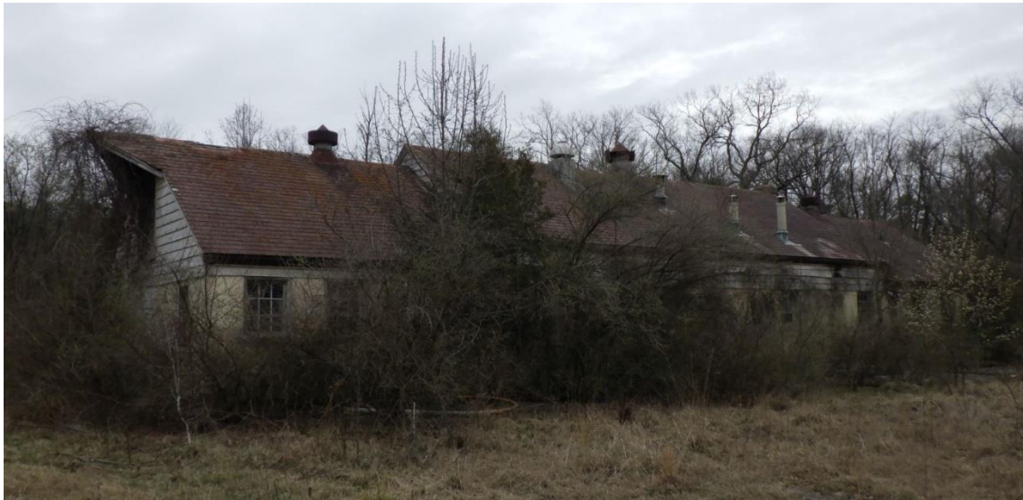
Figure 8-34: Building 543, facing southwest, location shown on Appendix A, Figure 4
