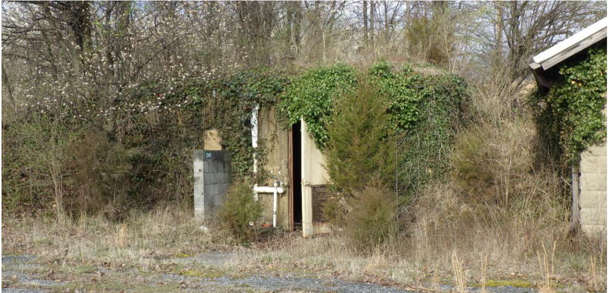
Figure 8-4: Building 41, facing southwest, location shown on Appendix A, Figure 2
