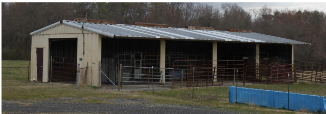
Figure 8-8: Building 435 – View from southwest, location shown on Appendix A, Figure 3
