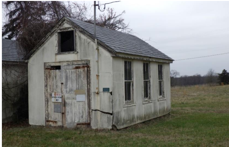
Figure 8-52: Building 1053 facing southwest, location shown on Appendix A, Figure 3
