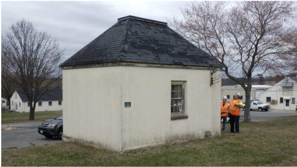
Figure 8-41: Building 1183 – Facing northeast, location shown on Appendix A, Figure 3
