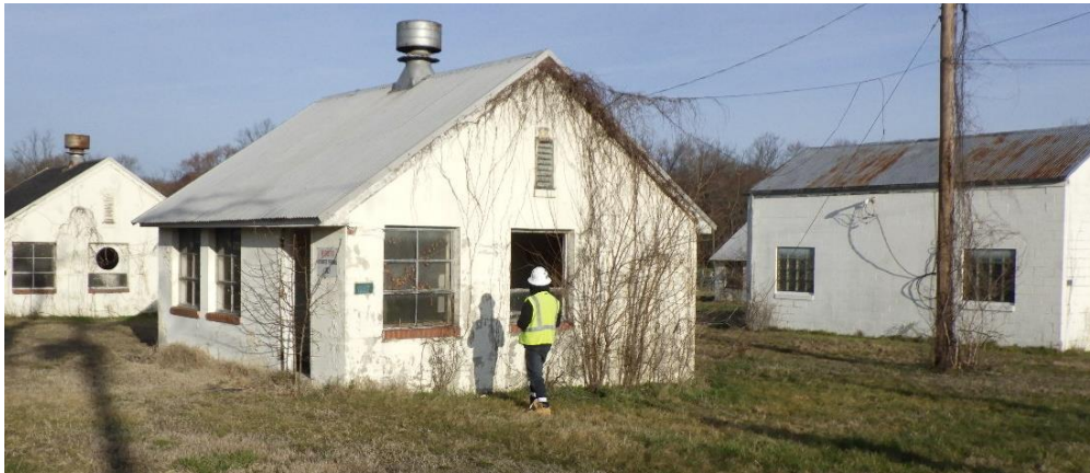
Figure 8-42: Building 1287 – Facing west, location shown on Appendix A, Figure 3
