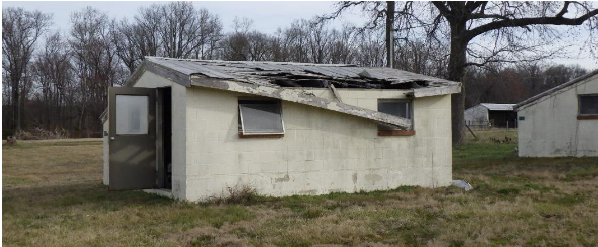
Figure 8-45: Building 1328 – Facing north, location shown on Appendix A, Figure 3
