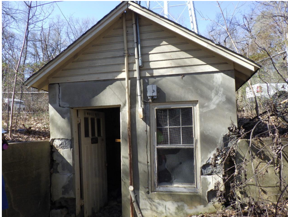
Figure 8-7: Building 287, facing west, location shown on Appendix A, Figure 3
