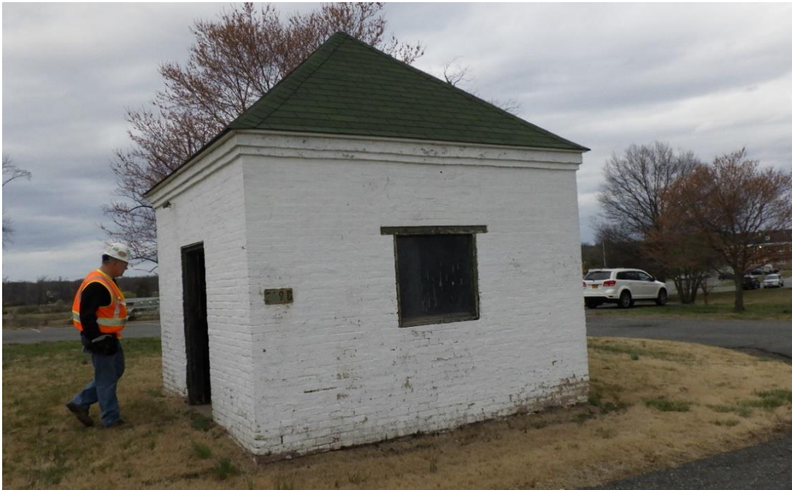
Figure 8-6: Building 209B, facing north, location shown on Appendix A, Figure 3
