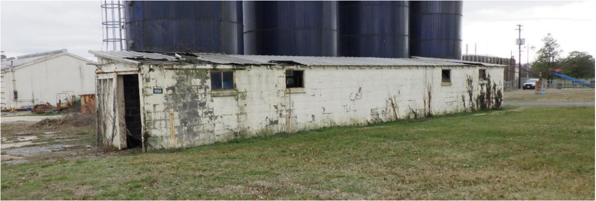
Figure 8-2: Building 166A, facing southwest, location shown on Appendix A, Figure 3 ACM
