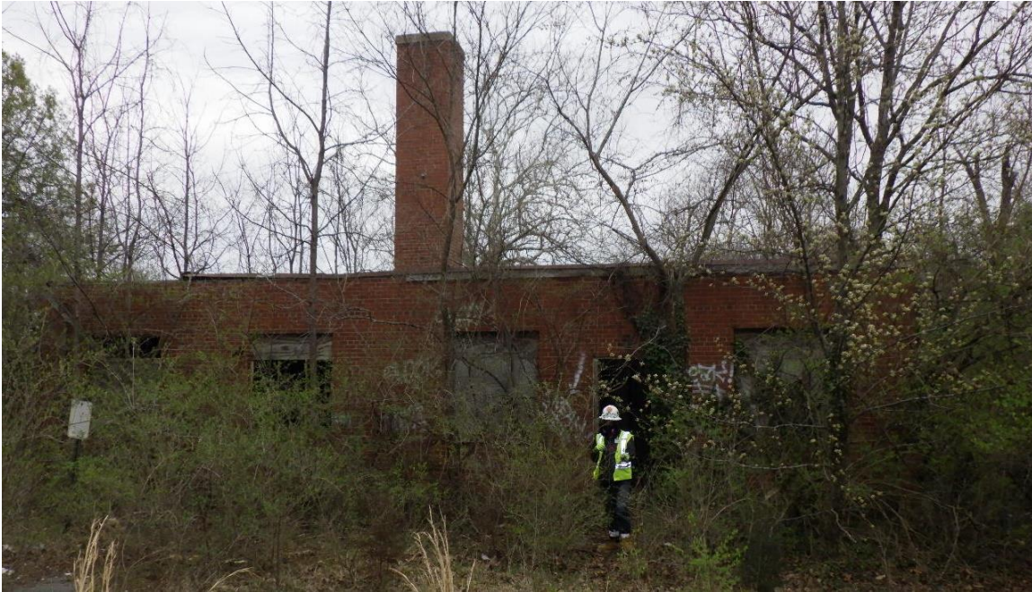
Figure 8-8: Building 85A, facing east, location shown on Appendix A, Figure 3
