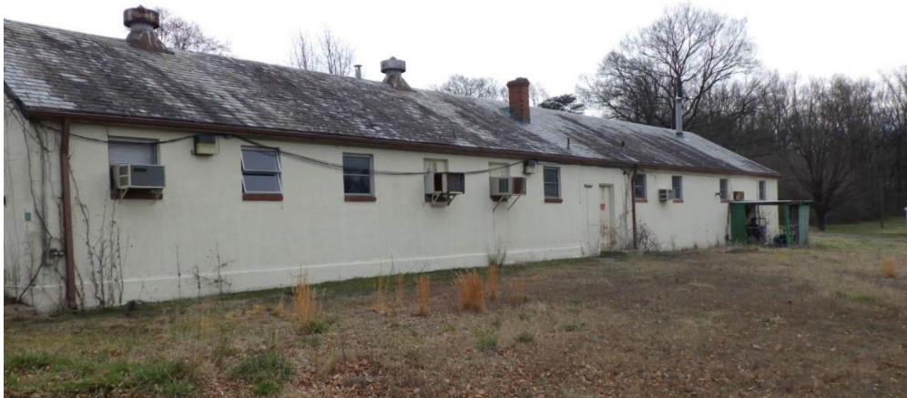
Figure 8-38: Building 1100 – facing southeast, location shown on Appendix A, Figure 3
