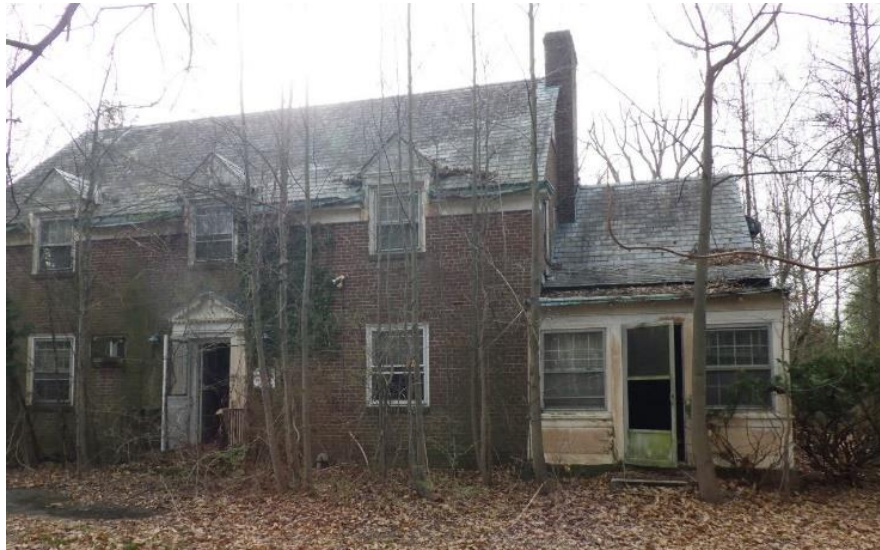
Figure 8-56: Building 1070 facing south, location shown on Appendix A, Figure 3
