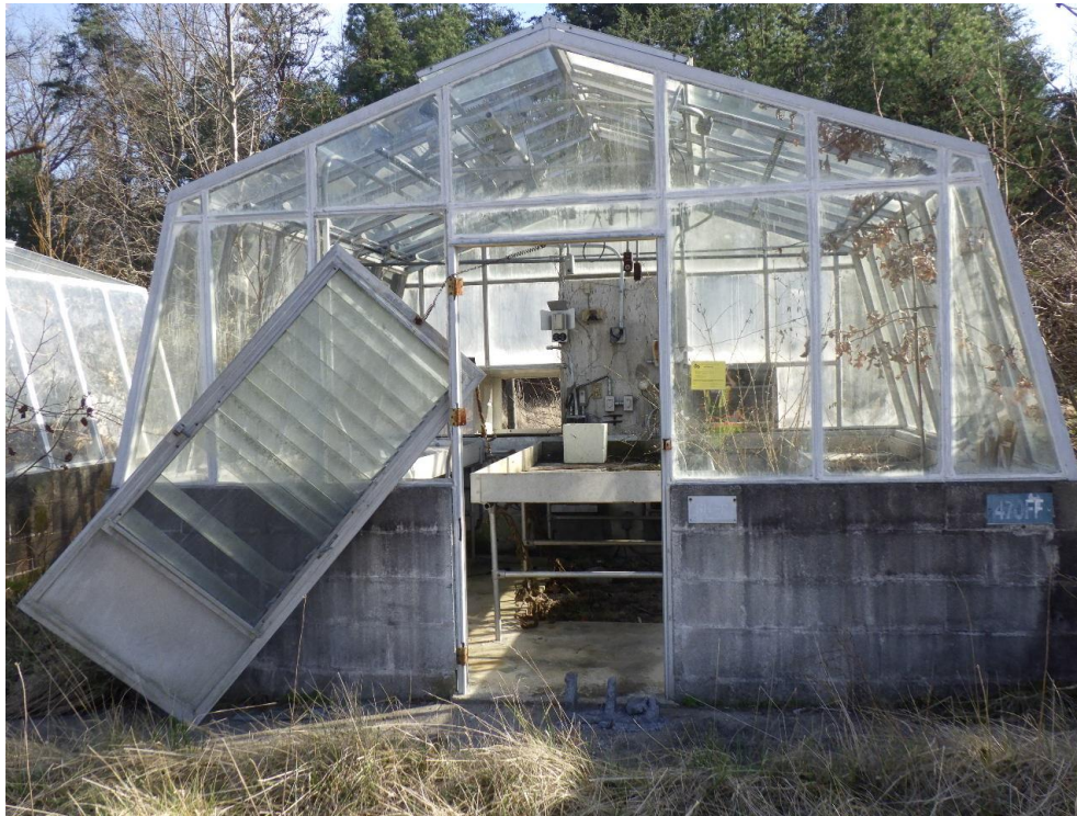
Figure 8-17: Building 470FF, facing south, location shown on Appendix A, Figure 3
